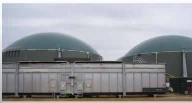
Two push floor dosing feeders, each with a MULTIMix, ensure that the digesters are continuously filled.
