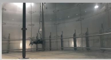
The stainless steel pre-storage tanks are equipped with a stainless steel floor.
